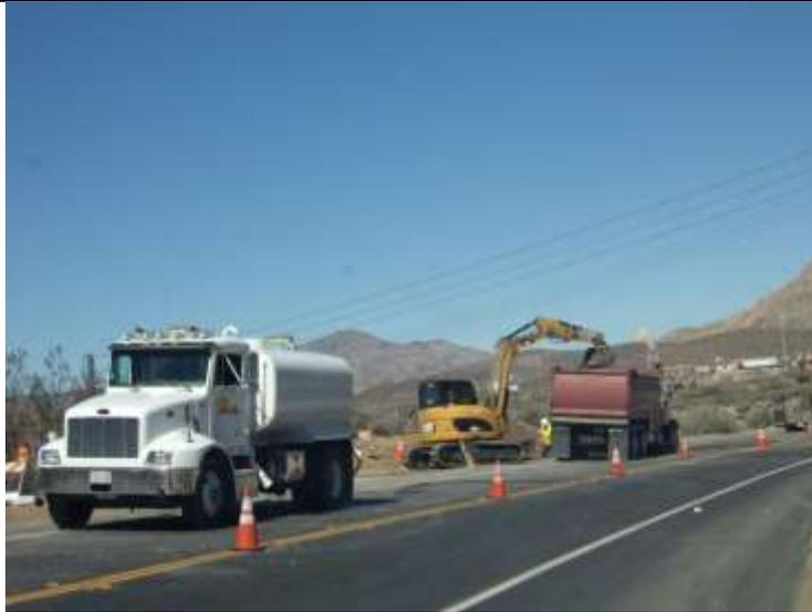
**Photo 3:** Water trucks were on site to suppress dust emissions during curb work at SP-91 in compliance with MM-BIO-4a and MM-AQ-1.
