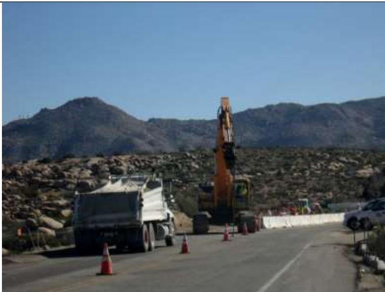
**Photo 2:** In accordance with MM-BIO-4a and MM-AQ-1, crews were observed covering spoil loads leaving Section 3 of the underground alignment.
